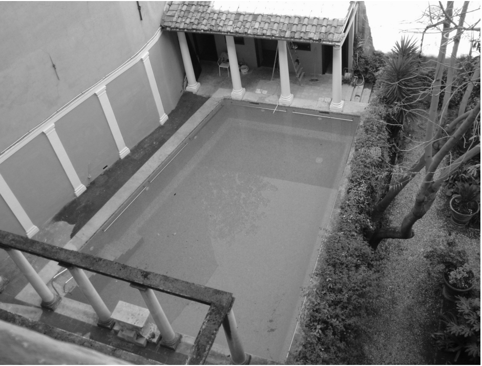
The restored and re-equipped Tank.
