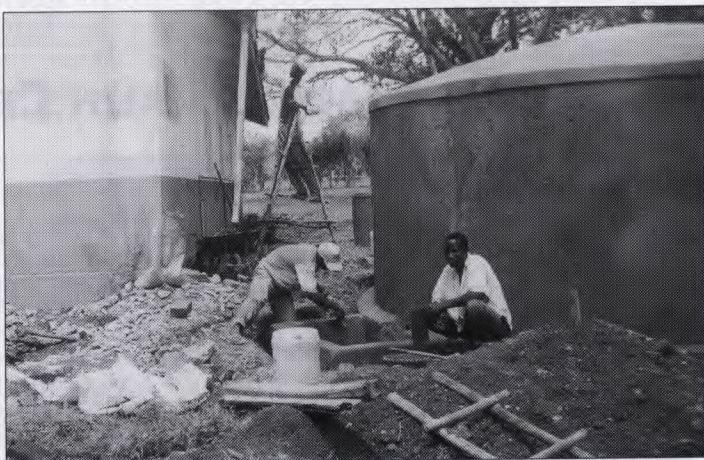
Final touches – the tap is fitted so that we can get the water!
