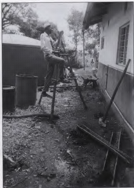
Putting up the new guttering.
