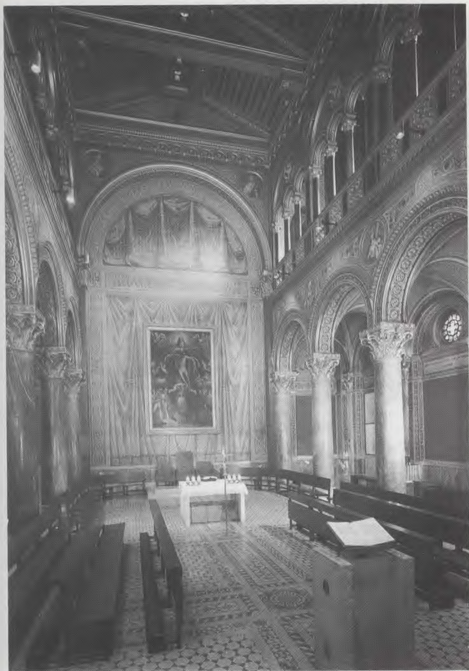
Interior of the Main College Church.
