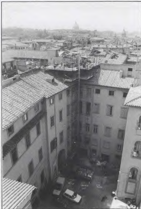
Repairs to the College roof.
