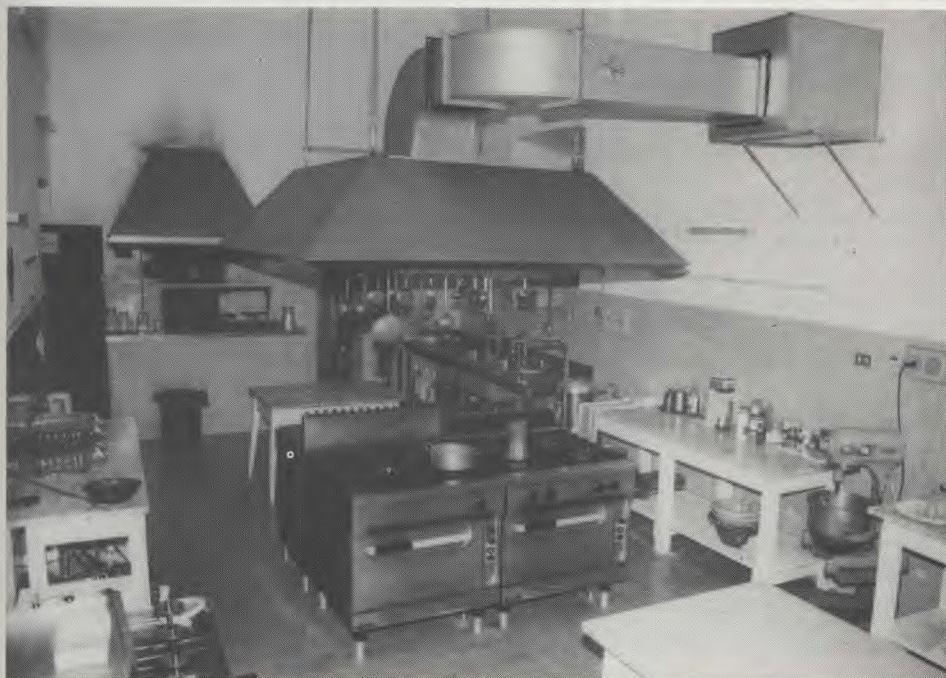
Villa Palazzola: the modernised kitchen
